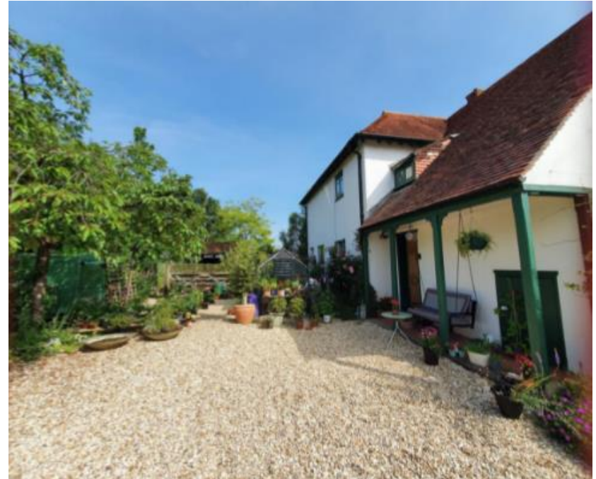
VIEW TO THE SOUTH-WEST WITHIN SITE – LOCATION OF PROPOSED ACCESS TRACK
