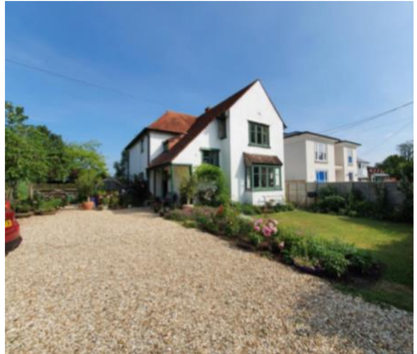
FRONT OF PROPERTY
